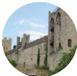
WALLS OF PIRAN
