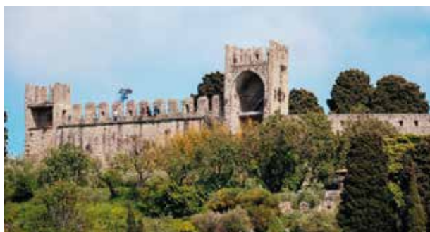
THE CITY WALLS OF PIRAN
